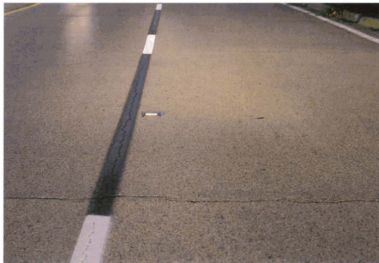
Roadway markers shine when struck by headlight beams to help drivers see the driving lane at night.
