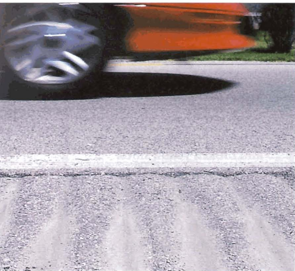
This type of rumble strip will let you know when you have wandered off the roadway.
